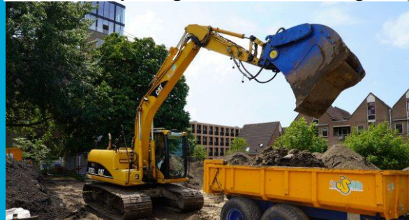
Crane drive train converted to Hydrogen Fuel Cell Electric
